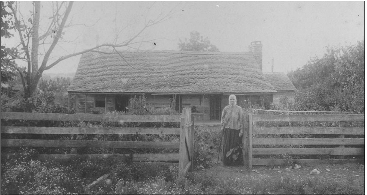
The Morton House, where the Borden Family and their neighbors waited out the Battle of Prairie Grove in the cellar. Courtesy Arkansas State Parks.
