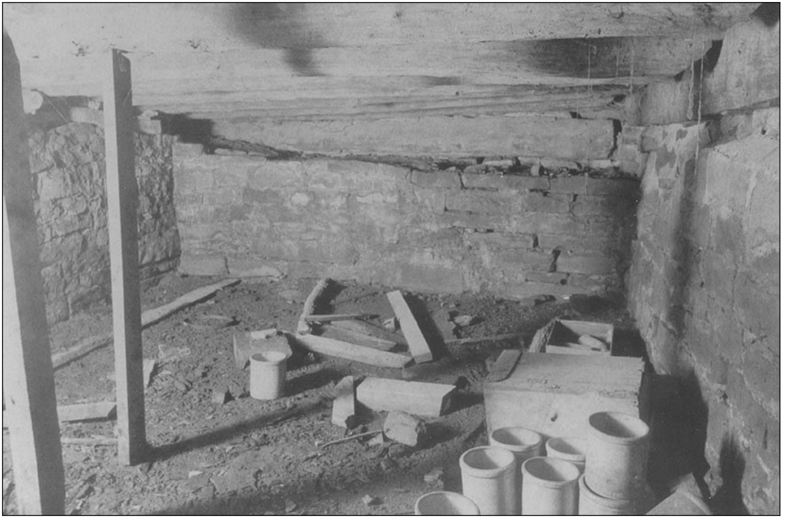
The Morton House Cellar, Courtesy Arkansas State Parks
