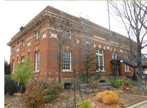
From top: James E. M. Barkman House, Arkadelphia, Clark County, NRHP 3/8/74; Spring River Bridge, Mammoth Spring vic., Fulton County, NRHP 1/22/14; Old U.S. Post Office, Fayetteville, Washington County, c. 1911, NRHP 8/27/74.
