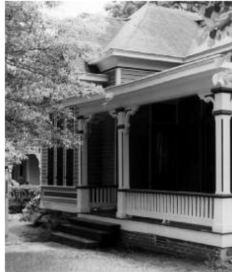
Character-defining features of a porch should be preserved. These include balustrades, columns, brackets and steps, as well as foundations and flooring materials.
