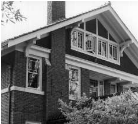
Window frames, brackets, molding and strapwork are examples of architectural features that contribute to the historic significance of a property which should be preserved.
