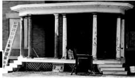
Preserve original porch features. Patch and repair significant features rather than replace.
