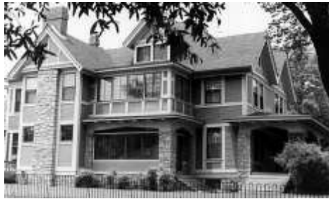
Decorative clapboard siding, multi-paned windows, chimney trim and a hooped metal fence are among the design details that contribute to the character of this property.
