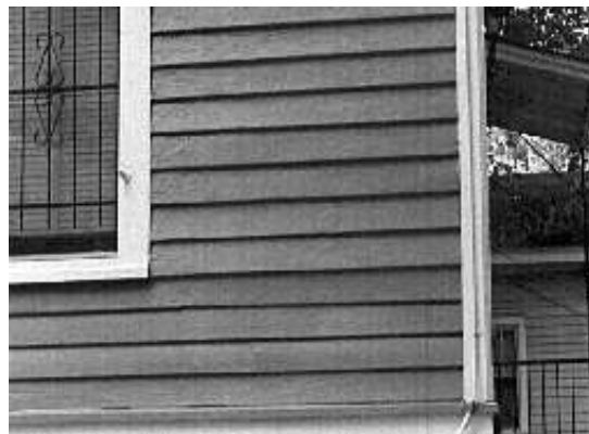
Wood is a typical Little Rock siding and is an appropriate material.
