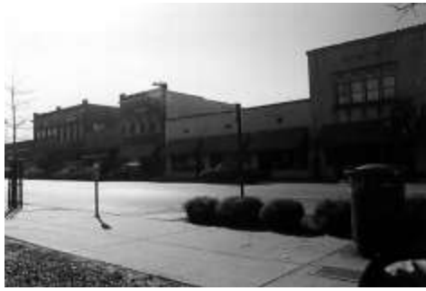
That portion of Main Street north of 19th Street, zoned "O," originally developed in a traditional commercial storefront context, where buildings are rectangular and aligned at the sidewalk edge.
