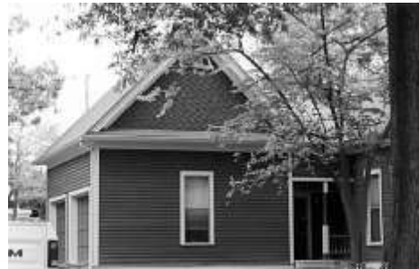
A new porch serves as the connector in the photo above, linking the new construction with the original.
