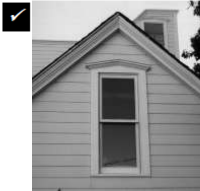
Match a replacement window to the original in its design.
