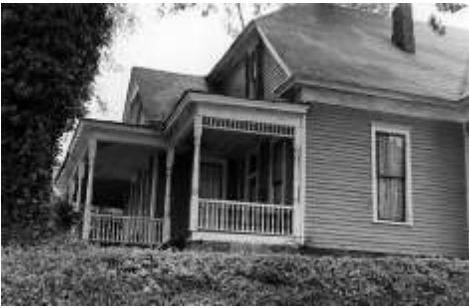
Preserve an original porch. Maintain the basic porch structure as well as its distinctive trim features.
