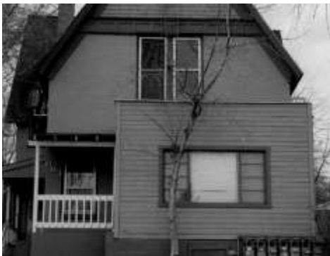
Do not construct a new addition that will hinder one's ability to interpret the historic character of the building or structure. This addition obscures the front porch, for example, and is inappropriate.
