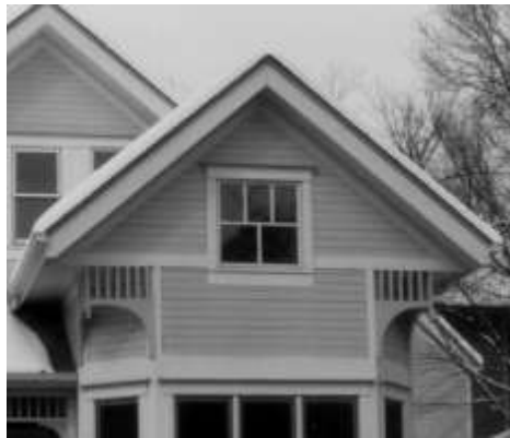
Contemporary interpretations of trim details and window moldings can provide visual interest while helping to convey the fact that the building is new.
