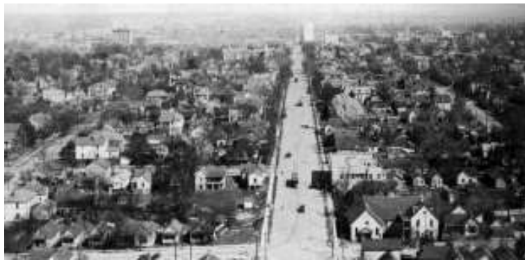
An early photograph from the Capitol, looking east toward downtown Little Rock illustrated the residential character that this street once had. The few surviving houses from this period are important historic resources that form a link to this part of the city's past.
