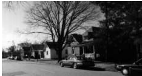
Several blocks of Little Rock's historic housing stock exist within the Capitol Area boundaries.
